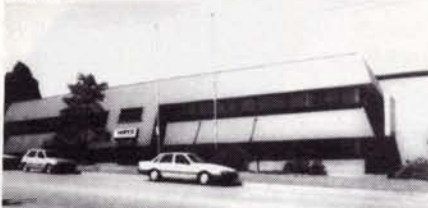
Mote Kennett new factory at Rydalmere, NSW.
